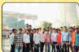
Mahatma Gandhi Thermal Power Plant, Jhajjar
